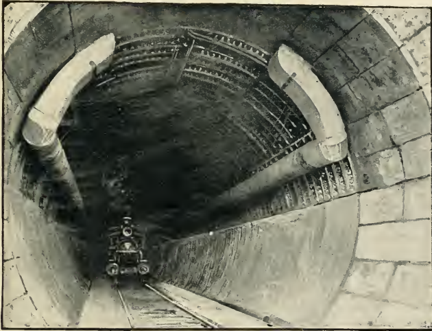
VENTILATING DEVICE, FOR REMOVING SMOKE.
